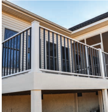
Multiple Color Rails and Balusters
